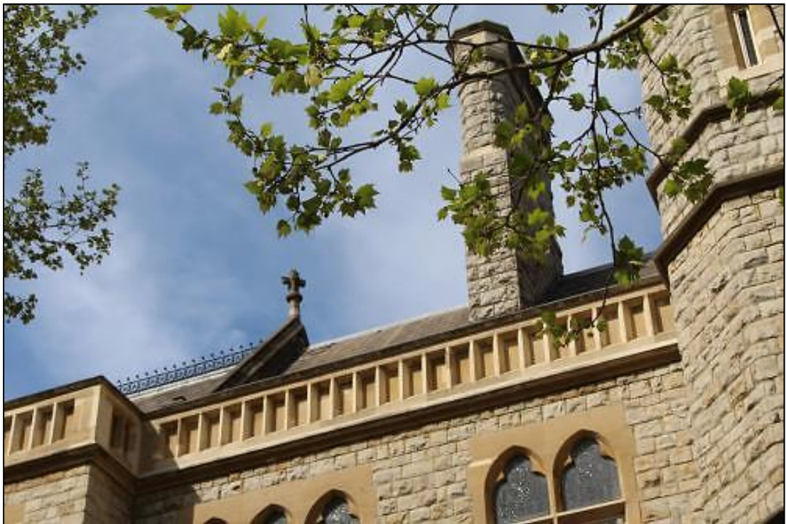
Photo 10: Roof and gable junction between phases B (left) and C (right).
