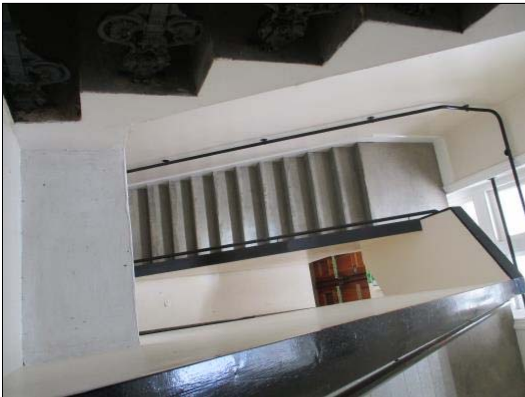
Photo 57: View of dog-leg stairs to south-east corner of Jones' original building. These lower flights were inserted during the later work to create a continuous flight of stairs in this area.
